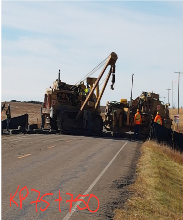
9. Bending Machinery/ Highway crossing – Location – 75km+750 - Oct 18, 2017
