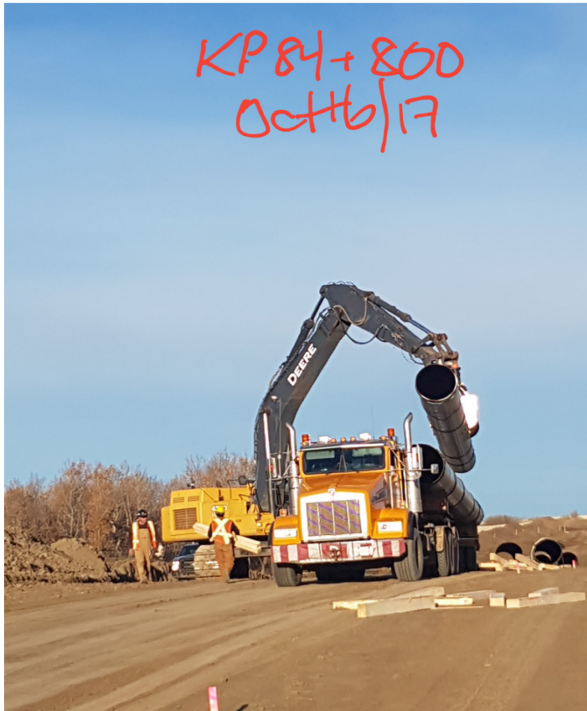
1. Stringing Crew –Location 84km+800 – Oct 16,2017
