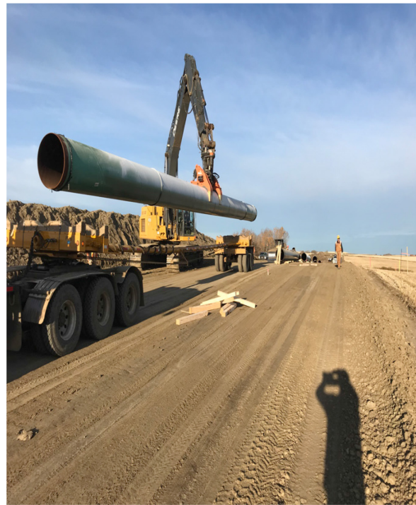
4. Stringing crew – Location 84km+800 – Oct 16, 2017
