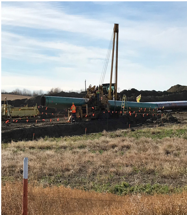
11. Bending Crew – Location – 75km+975 – Oct 18, 2017
