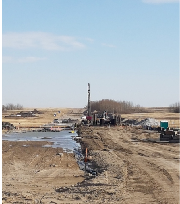
6. Driven Piles – Location 97km+200 – Oct 17, 2017
