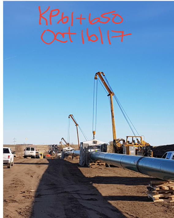
2. Welding Crew – Location 61+650 – Oct 16, 2017
