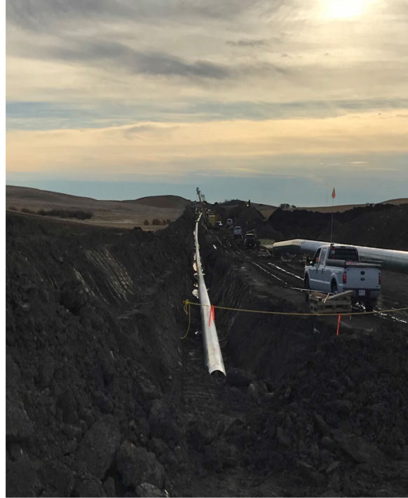
14. Laying in pipe – Location 29km+50 – Oct 19, 2017
