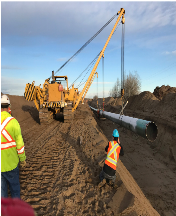
15. Welding in ditch – Location – 21km+600 – Oct 19, 2017
