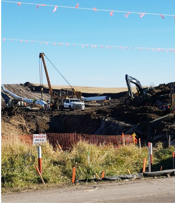
5. Boring – Location 36km+100 – Oct 16, 2017
