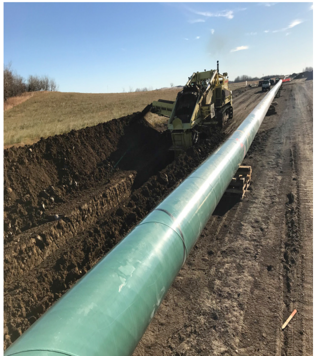
12. Ditcher – Location – 32km+450 – Oct 18, 2017
