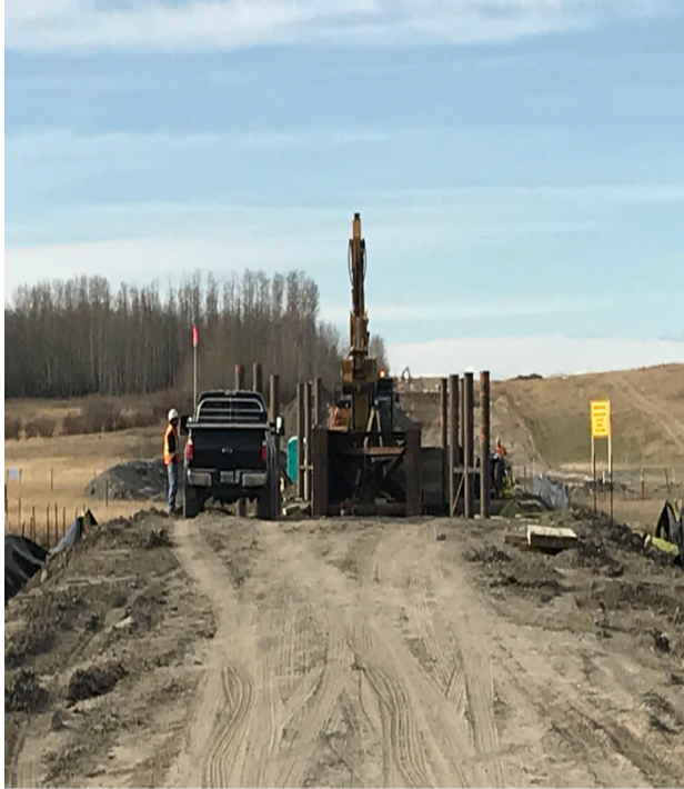
13. Bridge installation – Location 97+600 – Oct 19, 2017
