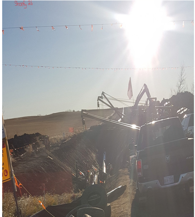
10. Laying pipe – Location Shoofly 26 – Oct 18, 2017
