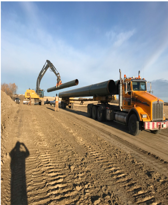
3. Stringing Crew – Location 84km+800 – Oct 16, 2017
